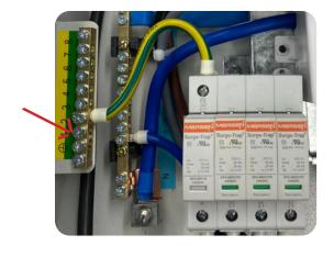
9) Attach the TPN front cover ensuring that the SPD goes through the window cut-out provided on the lid. Apply the labels to specify the MCB and SPD.
