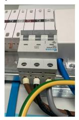
7) Connect the SPD to the Earth Terminal. Earth wire: PE (SPD) to Earth Terminal
