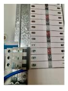
2) Ensure that the SPD cartridges are in the correct orientation (PE on top). If not, remove SPD cartridges from holder and replace. Ensure that the correct SPD module (Earth) is installed at the correct part of the holder.
